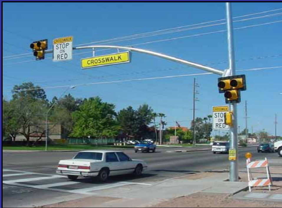
HAWK Signal in City of Tucson, AZ
